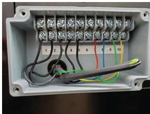
Figure 1: Remote contact terminal box with cover removed
